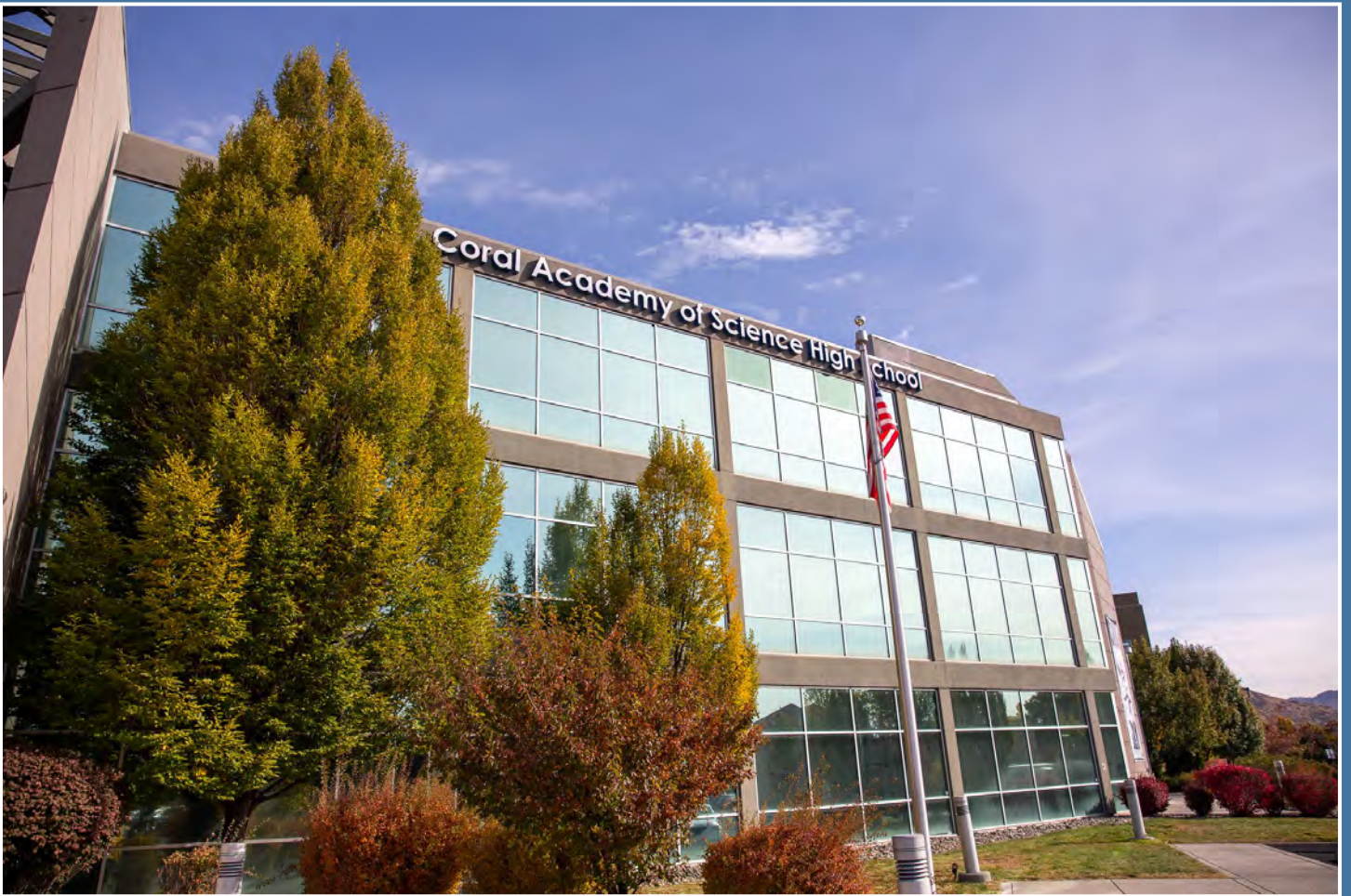
Above: The High School Facility located at 6272 Neil Road.
