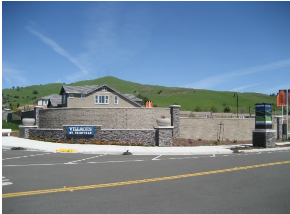
Project signage on Clay Bank Road at Gulf Dr.
