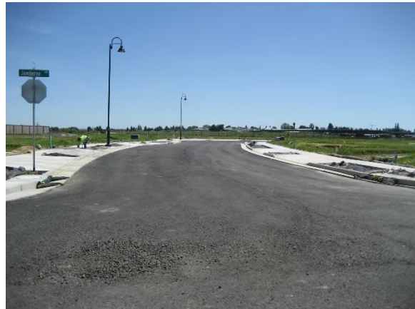
Looking south along Retreat Way in Unit 4 (final asphalt layer to be completed by Tri Pointe)
