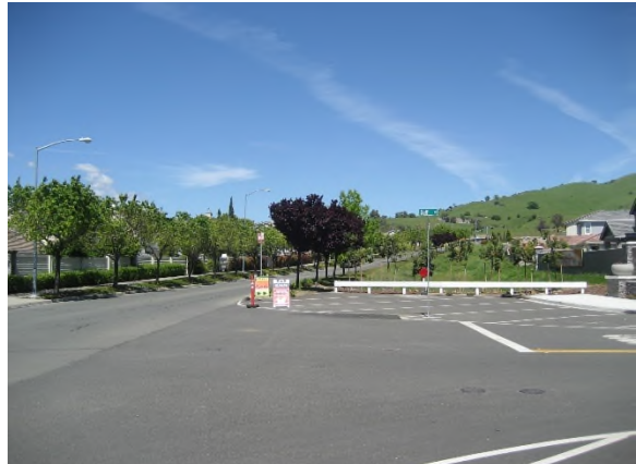
Looking north on Clay Bank Road at Gulf Dr. (future widening to be completed by non-subject properties)
