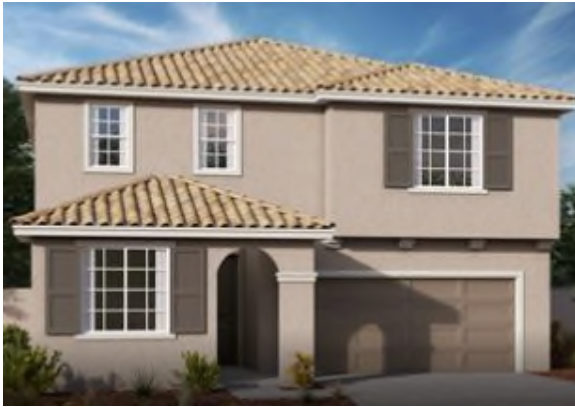
Comparable 3 – Montera by Richmond American Exhibit from Builder website; models under construction
