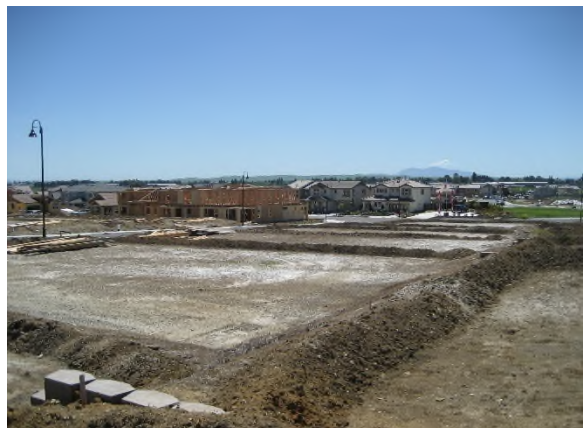
Looking south across Unit 1 toward Unit 3
