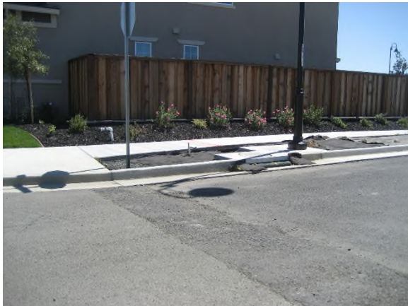
Final asphalt layer not yet completed west of Horizon Circle in Unit 4 (to be completed by Tri Pointe)
