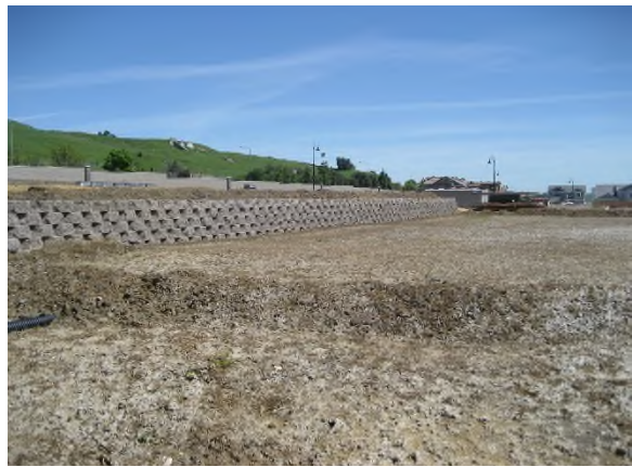
Lot terracing and leveled building pads in Unit 1
