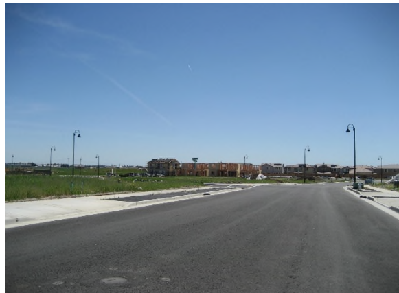
Looking south along Inspiration Dr. (Unit 3)
