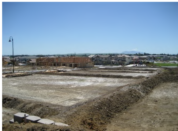
Looking south across Unit 1 toward Unit 3
