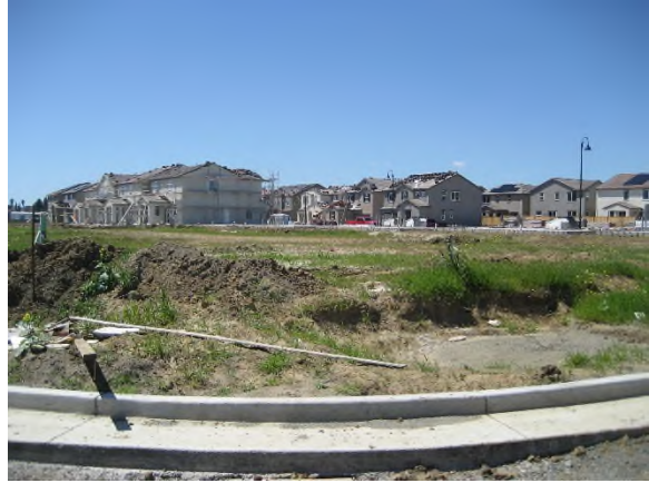
Looking west across Unit 4 at homes under construction by Tri Pointe
