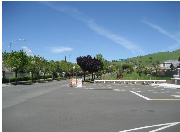
Looking north on Clay Bank Road at Gulf Dr. (future widening to be completed by non-subject properties)
