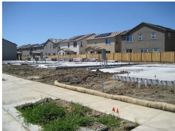
Homes under construction (foundations in foreground) and Substantially Completed homes (background) in Unit 4
