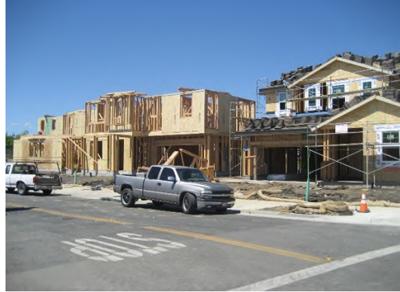
Homes under construction on Friendly Valley Ln. (Unit 3)
